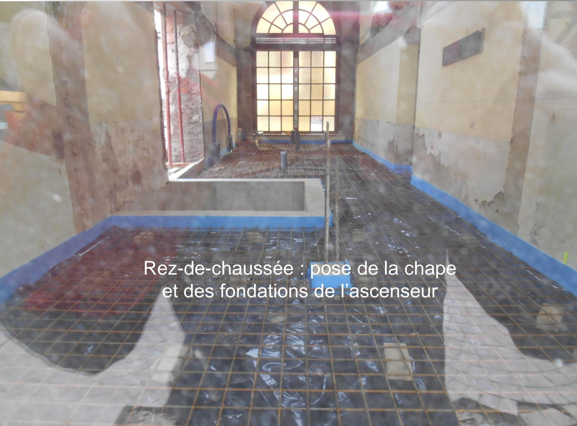
A photograph of a construction site on the ground floor. The floor is covered with a grid of steel reinforcement bars (rebar) laid out on a blue plastic membrane. A concrete foundation for an elevator is visible in the foreground. In the background, there is a large window with a semi-circular arch and a grid pattern. The walls are partially finished with yellow plaster, and some areas show exposed brickwork. A blue pipe is visible on the left wall.
